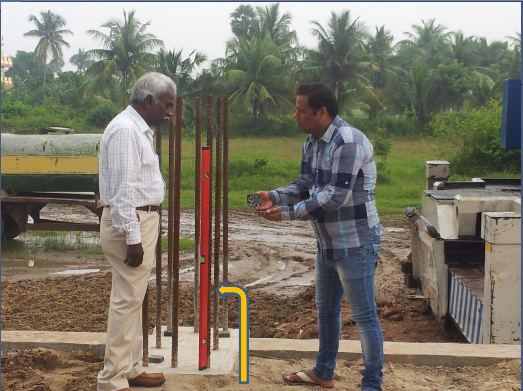
CHECKING LEVELS OVER PEDESTALS BEFORE ERRECTION OF COLUMNS
